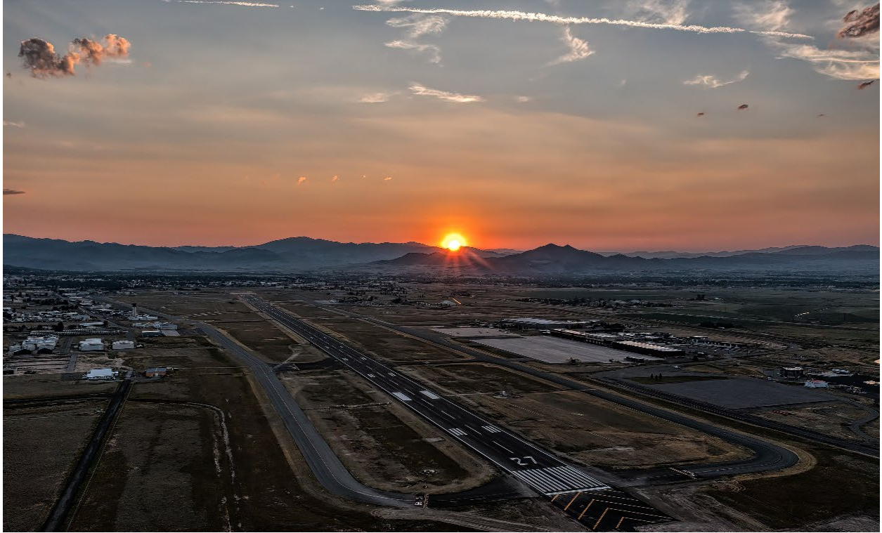
9,000' X 150' Primary Runway - Full Rehab Completed June 2021
