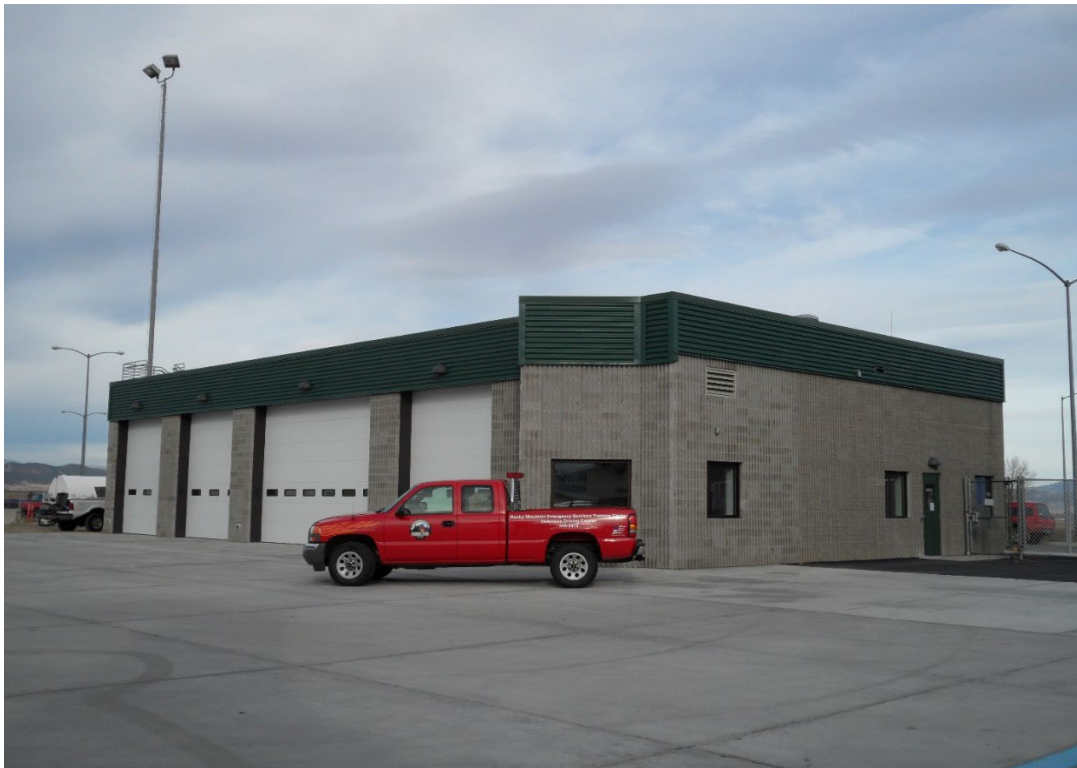
Fire Station #2 / Airport Operations Offices
